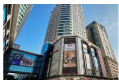
Ba Trieu Office Building
